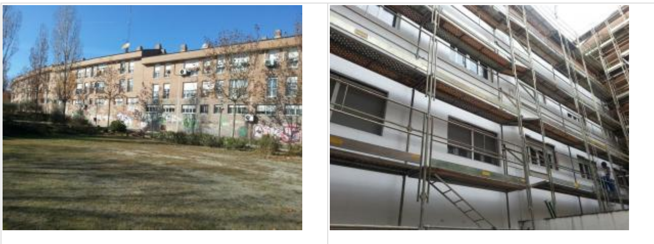
Figure 6. Renovation works "Oscar" building in San Sebastián de los Reyes (Madrid).
