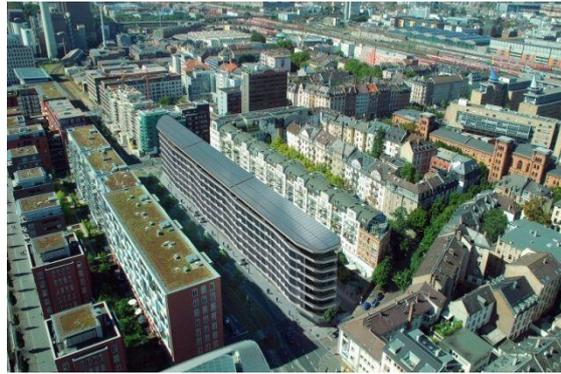
*Figure 2: The Solar Active House in the city centre of Frankfurt features a heat pump coupled to the sewage water and PV modules on the roof and the façade. (Source: HHS Architekten)*
